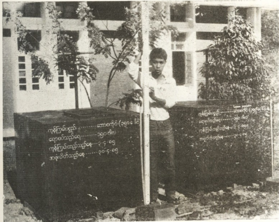
Fig 2. Digester of the Biogas Plant.
